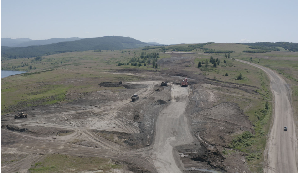
Ongoing construction of a new 10% grade mine haul road for First Mode's new Hydron Powered haul truck.
